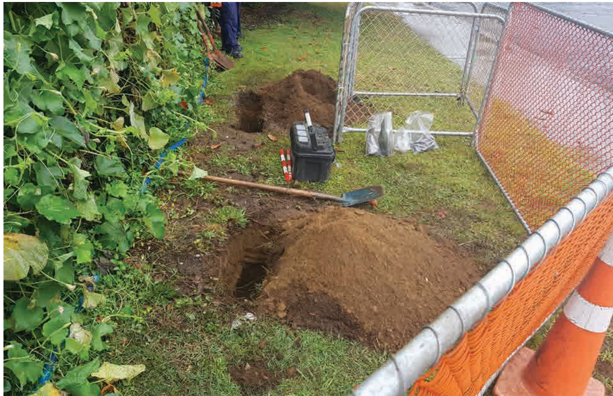
Figure 8. View east of two potholes where Feature 1 was exposed.
