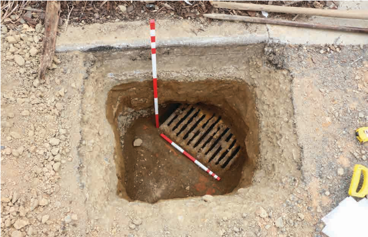
Figure 6. Decommissioned drain outside the Alpha Hotel. Photo scales = 0.5 and 1 m.
